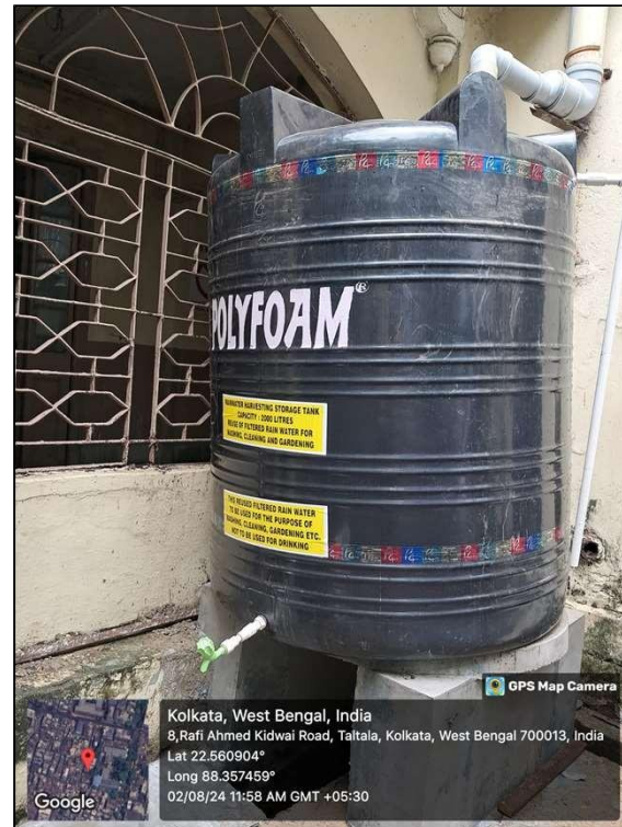
Rainwater harvesting units for rainwater storage and reuse
